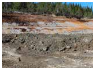
June 2013. The area that had previously been an open pit is now filled with waste rock, contaminated material and lime and has been covered over.
