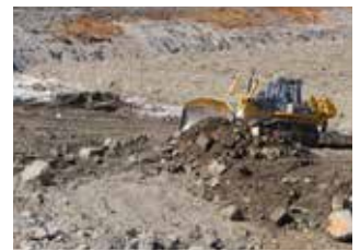
May 2013. The deposited material was covered with peat and a 0.5 m thick layer of till.
