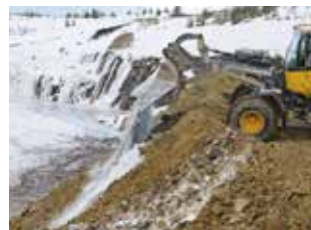
January 2013. Waste rock and material from the industrial area was deposited in the empty open pit. This work began in January 2013 and was completed in June 2013.
