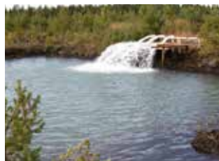
Kedträsk, September 2012. While draining the open pit, the water was limed a number of times. The water was collected in settling ponds so that the sludge could be dealt with and the water quality controlled.
