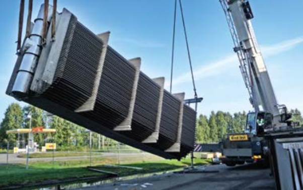
← Two cranes hoist a new evaporator heating surface.
