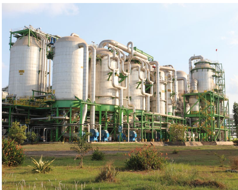
The evaporation plant at the OKI mill has 7+ effects and very high final dry solids for extraordinary overall energy efficiency.
