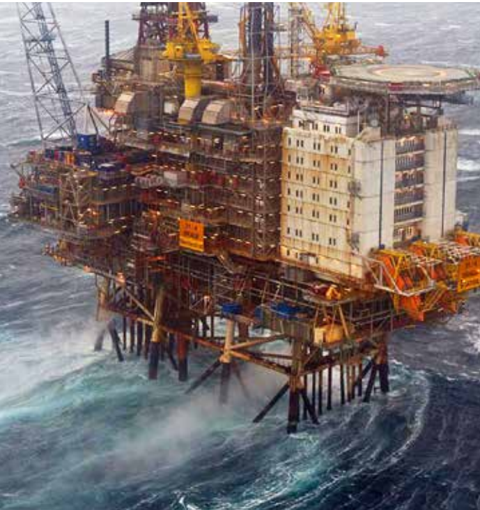
Brage in the North Sea is one of many Norwegian fields developed with a platform supported on a steel jacket. (Photo: Wintershall)
